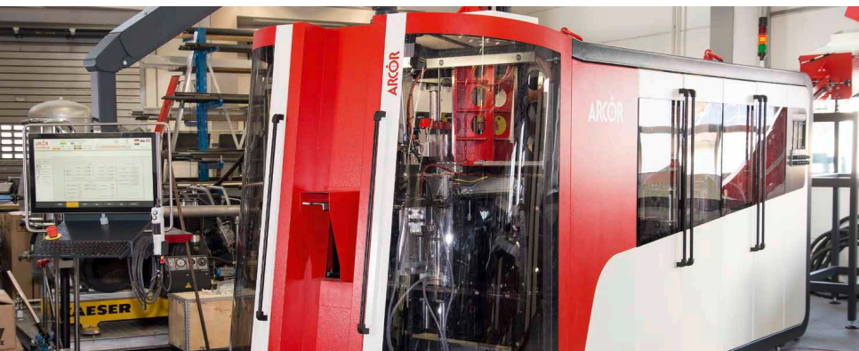
WAGO's EPSITRON® PRO Power Supply Unit powers the automation components in the control cabinet of a blow-molding machine.
