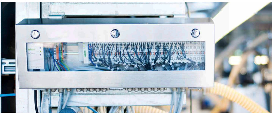
WAGO's EPSITRON® ECO Power Supply powers a machine data collection system for production.
