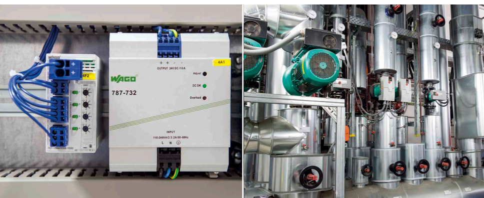
WAGO's compact 787-1664 Electronic Circuit Breaker provides reliable and precise overcurrent protection on the output side.
